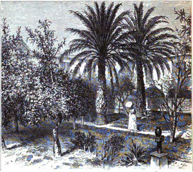
INTERIOR OF A LIMA DWELLING.
